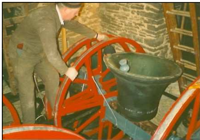
Trevor Bailey, the Whitechapel bell hanger ringing the 3rd from the wheel to adjust the clapper
