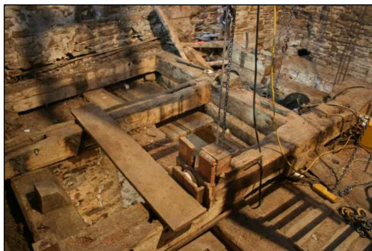
Sills of the 16 th /17 th Century five-bell frame standing on the older primary timbers
