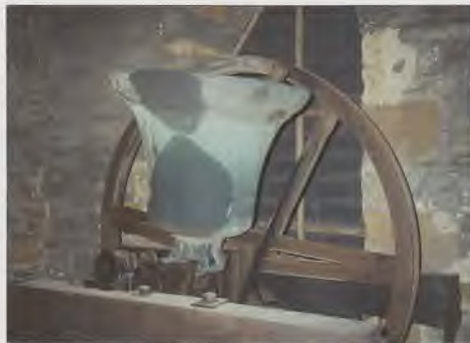
The bell at Castlethorpe . Back in action after a bolt tightening session.
